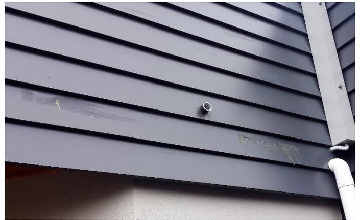
An extreme example of Resin Bleed on LOSP treated weatherboard.
